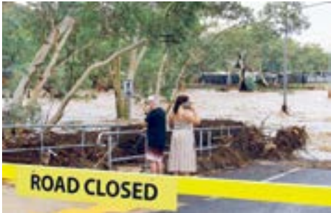
CLOSED: Debris caught on damaged railing at the closed Palm Circuit crossing. (534725)
