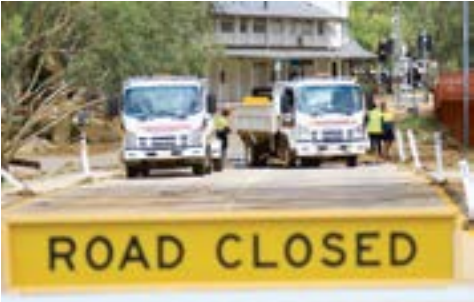
CLOSED: The closed Wills Terrace causeway as council workers repair damage to the road surface. (534725)
