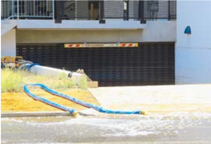
PUMPS: Pumps work hard to remove water from the car park of residential accommodation on South Terrace where around 20 cars were flooded. (534725)
