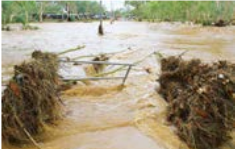
FLOTSAM: Debris washed down the river added to the damage caused to infrastructure. (534725)
