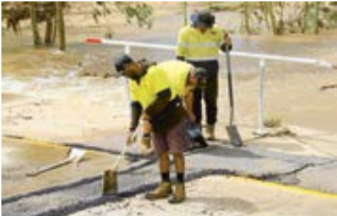
REPAIRS: ASTC workers make repairs to the road surface of the Wills Terrace causeway. (534725)
