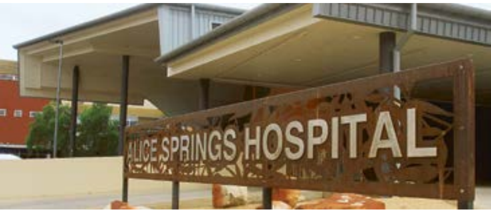
Exterior of the Alice Springs Hospital. (Phil Williams: 523750)
