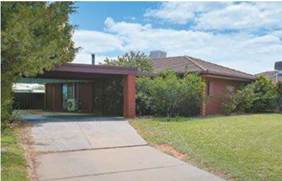
15 Etherington Drive, Mildura
