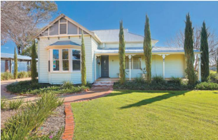
229 River Avenue, Merbein
