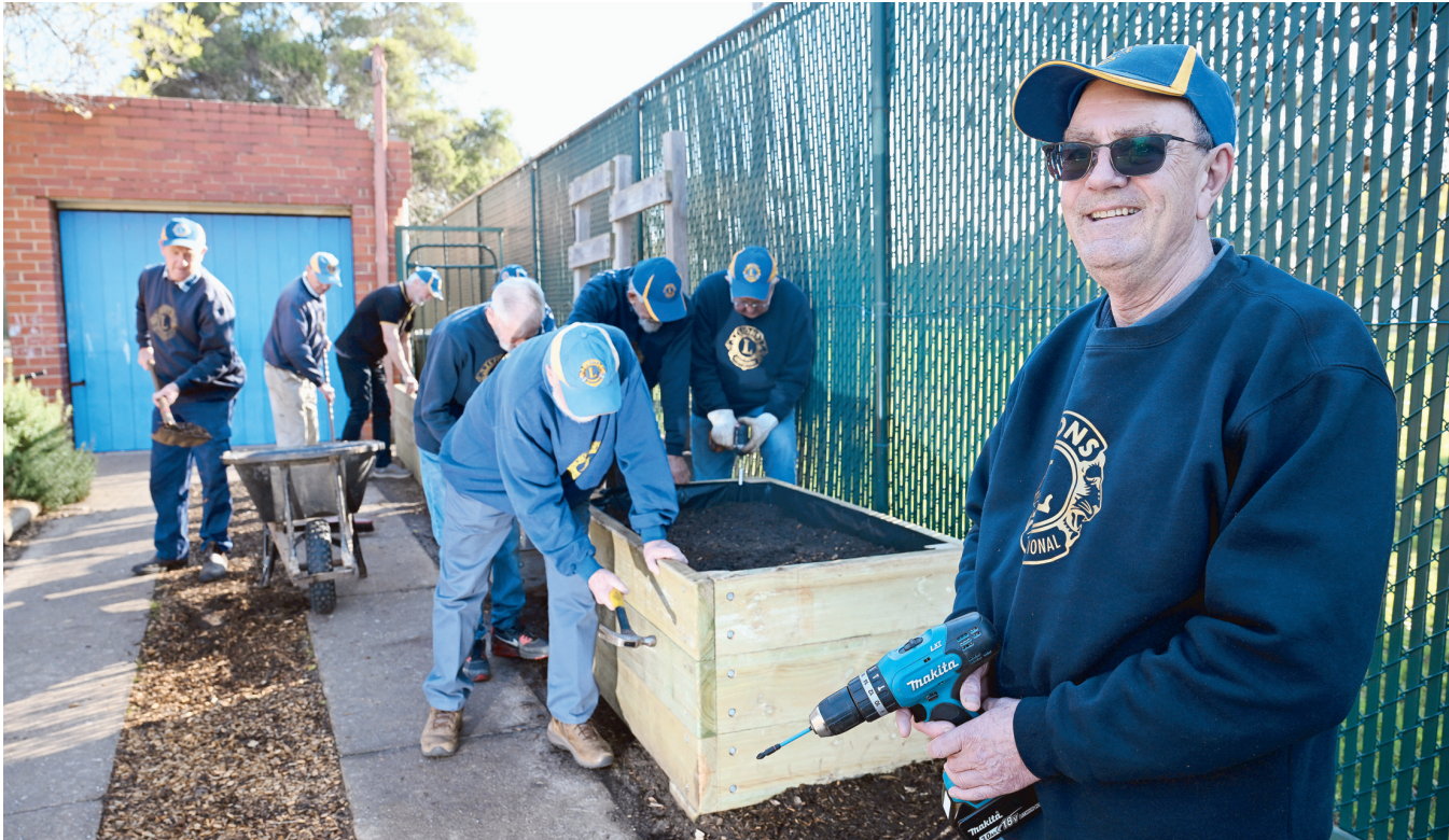
Lions Club president John Peebles and volunteers spent a frosty morning installing the new planter boxes at Young Street Kindergarten in Bacchus Marsh. (Damjan Janevski). 564403_03
