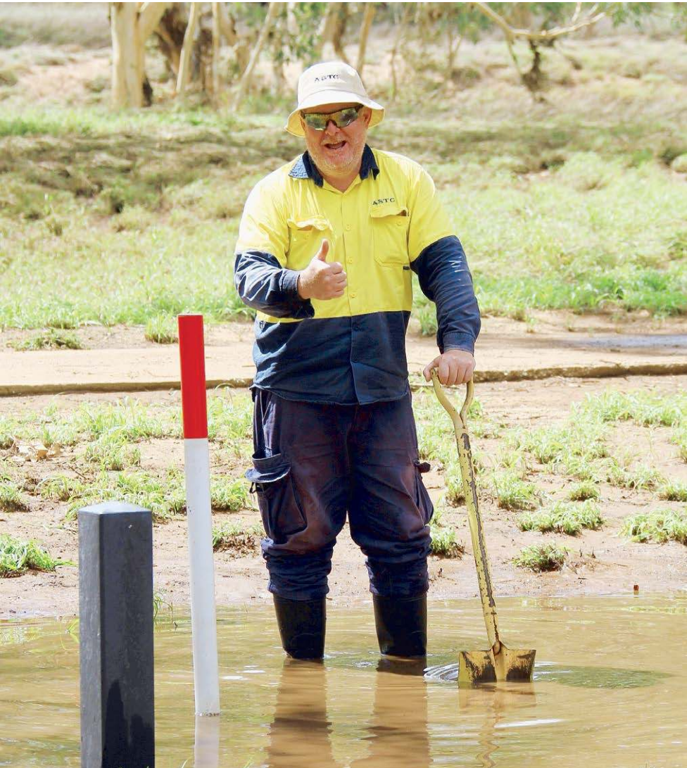
CLEAR: Council worker Ian Kelly knee deep in water as he clears a drain on South Tce. (Phil Williams: 534725)
