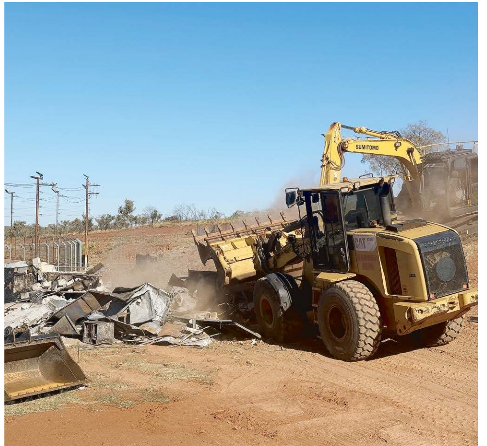
Volunteers turned out to a working bee to demolish the remains of the Speedway control tower and canteen following an arson attack three months ago.
