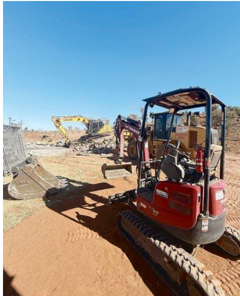
Local contractor Glen Barber from Barber Hire loaned his equipment to help clear the Speedway site.
