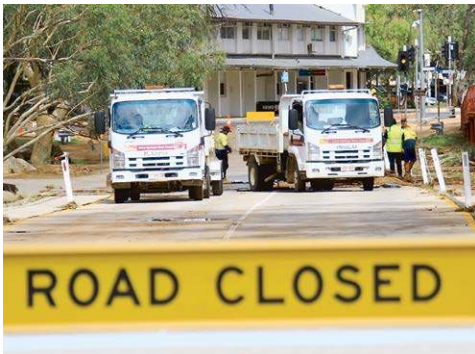
CLOSED: The closed Wills Terrace causeway as council workers repair damage to the road surface. (Phil Williams: 534725)
