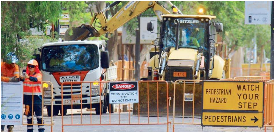
CONSTRUCTION: Todd Mall construction works. (Phil Williams: 531846)
