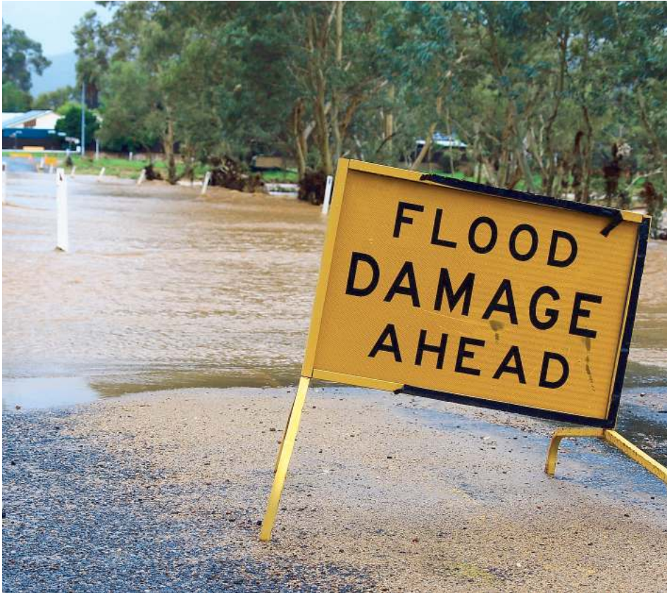
BOIL: The Todd River appears to boil as it races over the Wills Terrace causeway earlier this year. (Phil Williams: 537763)
