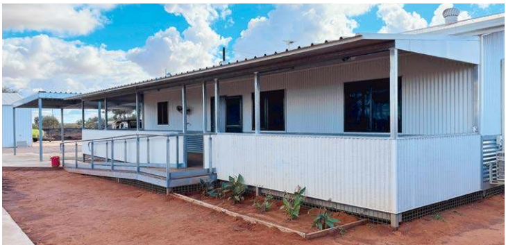
BASE: The office which replaces a shipping container at the new Aputula ranger base (Central Land Council)
