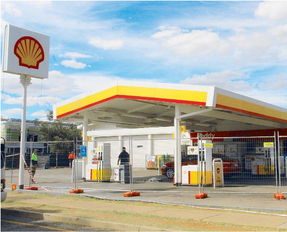
FENCED OFF: The Shell service station on Gap Road was extensively damaged after being looted during the Alice Springs riot. (Phil Williams: 550927)
