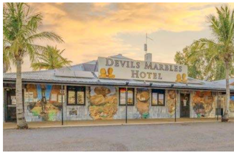
The Devils Marbles Hotel has declared it will no longer sell takeaway alcohol after it staff were injured and major damage caused in the latest break-in on 23 April.
