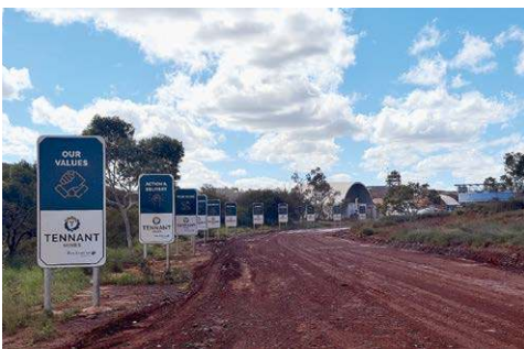
Tennant Mines' Central Processing Facility near the old Nobles Nob mine. "It makes sense to consolidate all of Tennant into one entity and eliminates the complexities of the joint venture agreement," he said.
