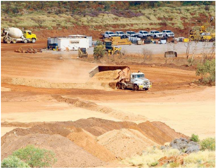
CONSTRUCTION: Early construction works at the Noble Nob Mine site in 2024.
