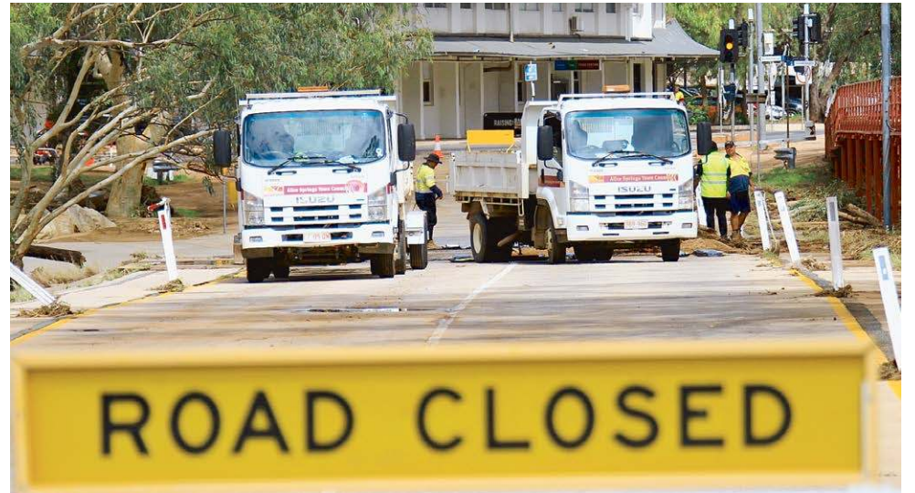
CLOSED: The closed Wills Terrace causeway as council workers repair damage to the road surface. (Phil Williams: 534725)
