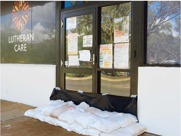
SANDBAGS: the Lutheran Care office sandbagged to prevent any further damage. (Phil Williams)
