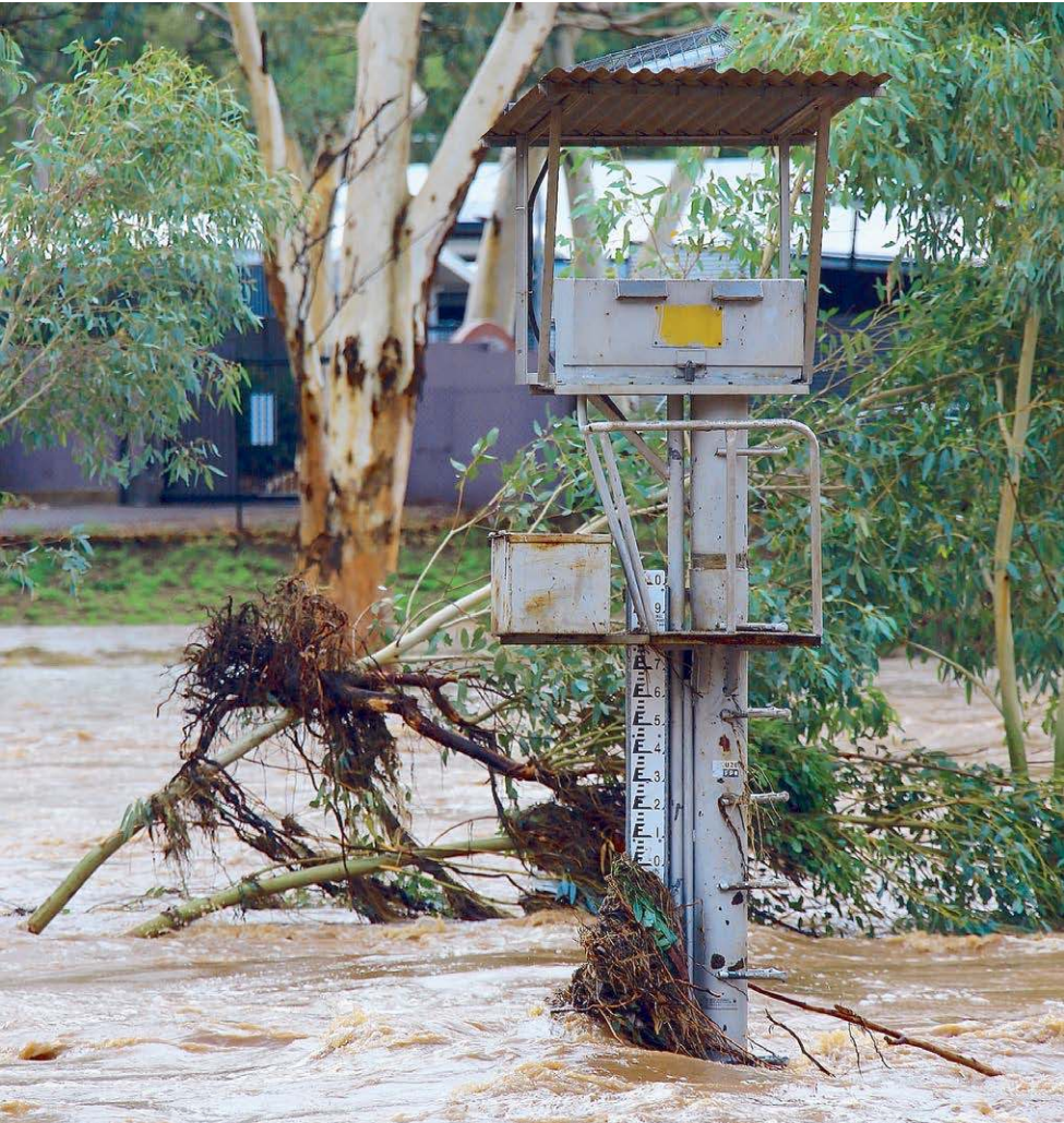
HEIGHT: Flood measuring equipment in the Todd River. (Phil Williams: 534725)
