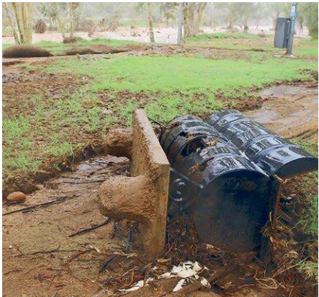
RIPPED OUT; A specially made park bench near the Wills Terrace causeway torn from it's foundation by the force of the water. (Phil Williams)
