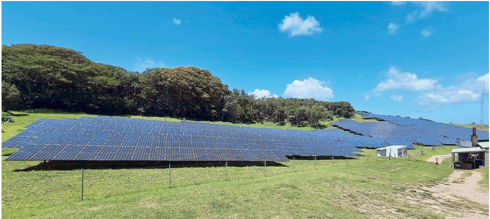
Commissioned in April 2021, the massive Hybrid Renewable Energy Project on Lord Howe Island delivered more than $1.5 million in diesel fuel cost savings in its first two years of operation, according to a 2024 review.
