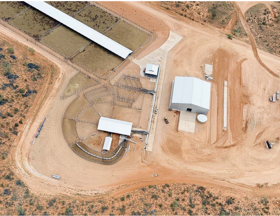
CATTLE: The newly completed transit yard.
