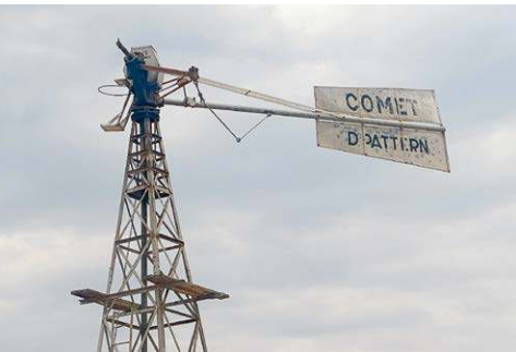
DAMAGE: The damaged tower of the Bonney Well windmill.
